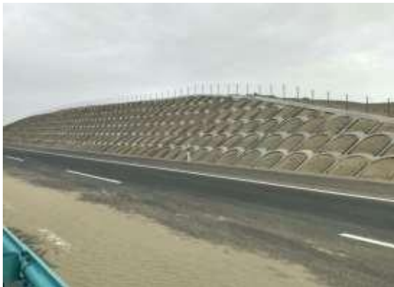
挖方边坡拱形骨架防护
